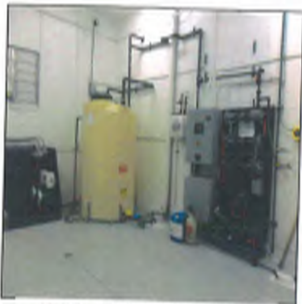
Fig. 54 – stand-by Miox system (not on line)
