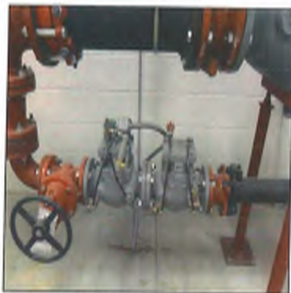
Fig. 29 - pressure reducer
