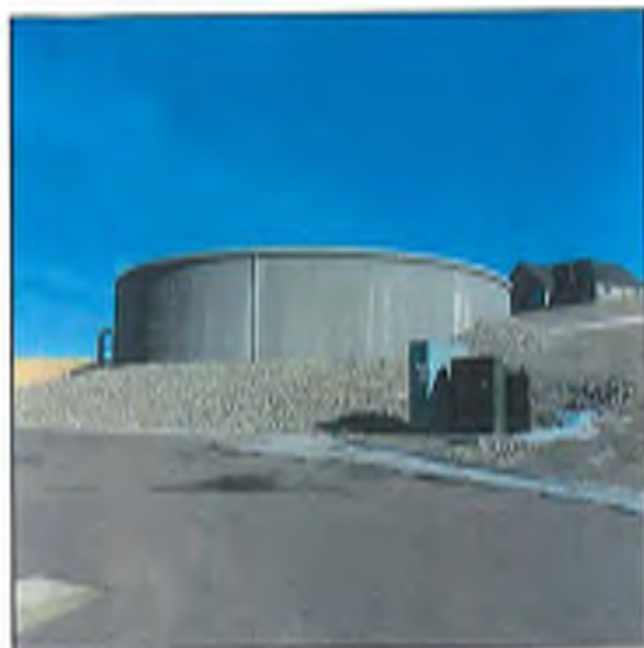
Fig. 49 – 2 million/gal storage tank (fed by well # 9 & 11)
