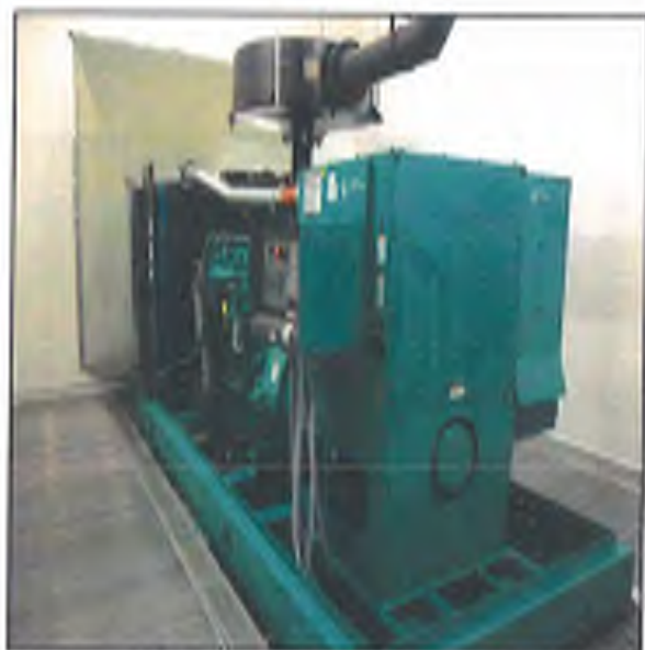
Fig. 63 – back-up generator
