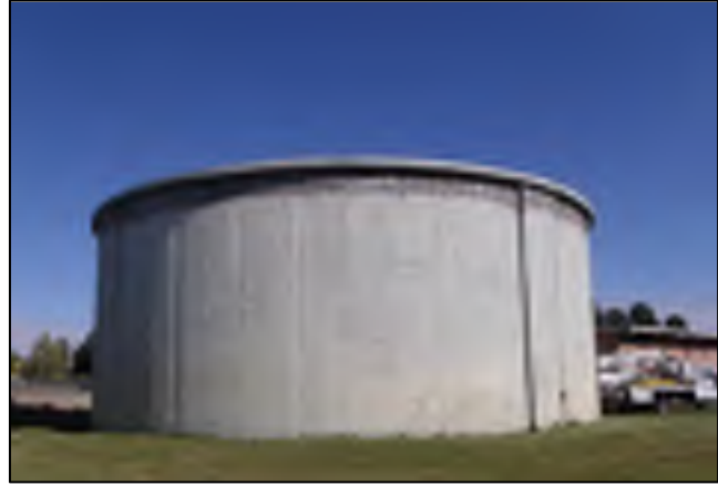
Ammon Well #6 Tank
