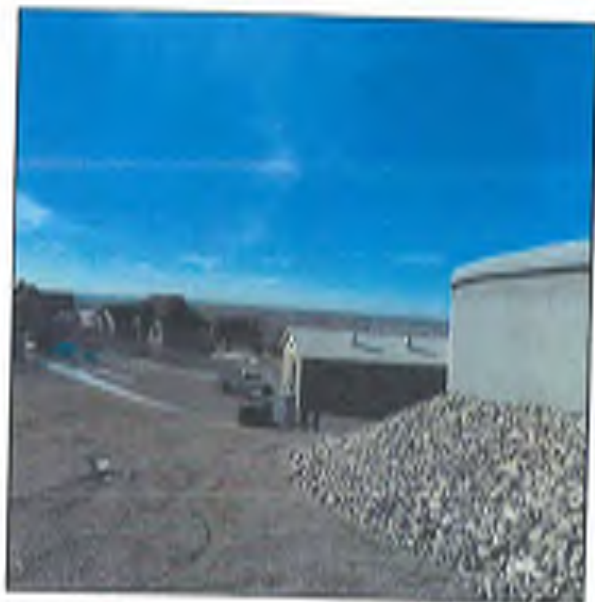
Fig. 56 – overall view of booster station and storage tank lot
