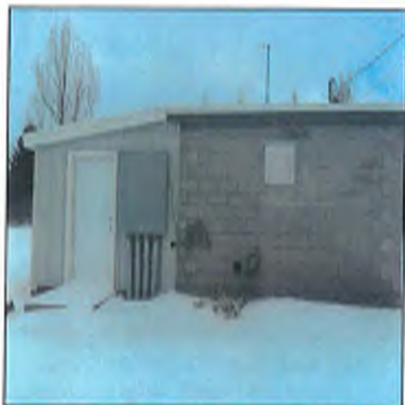
Fig. 1 – Well House # 5 (addition is for fiber optic equipment)
