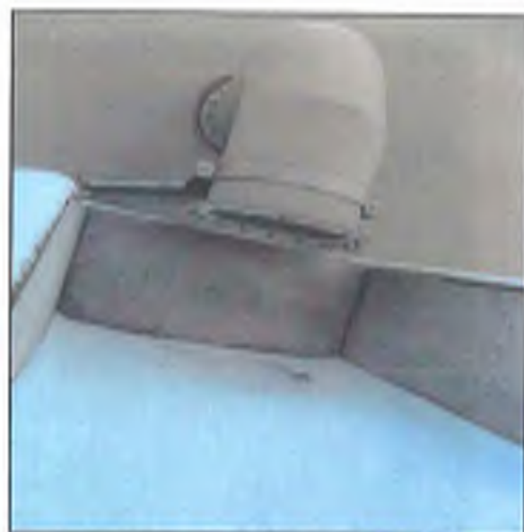
Fig. 16 – screened tank overflow
