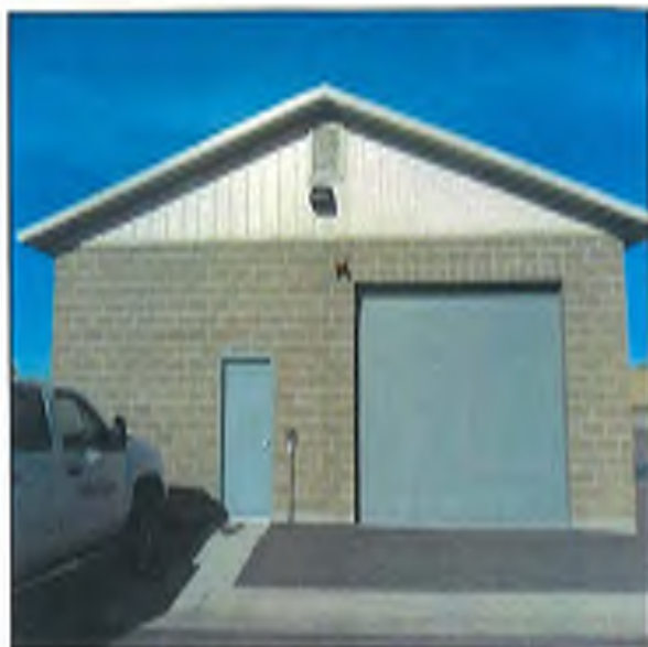
Fig. 50 – booster station building
